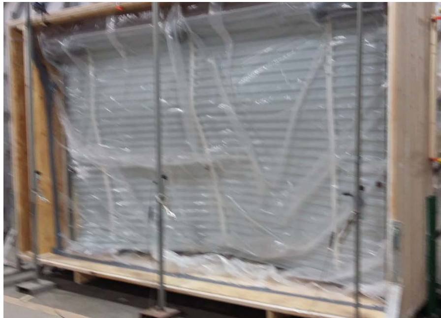
Photo No. 4 Interior View-Test Setup
