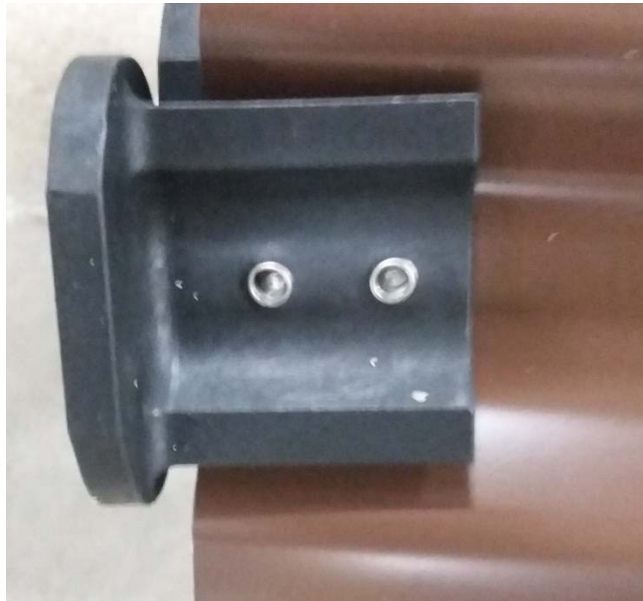
Photo No. 1 Wind lock
